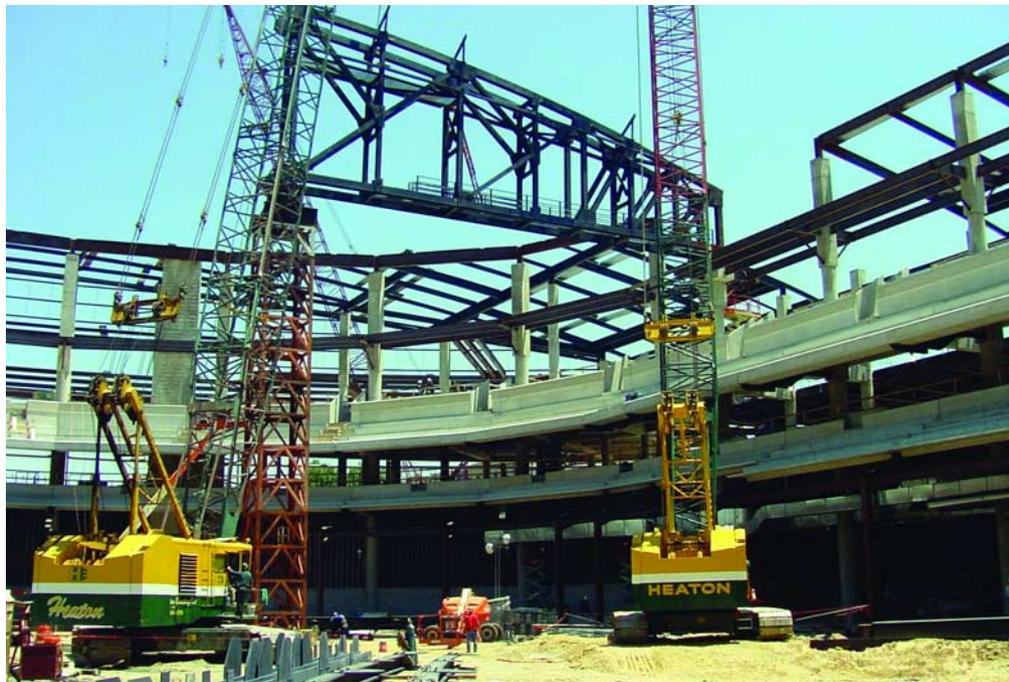
sense to have the truss bottom-chord elements serve double duty as rigging-grid beams. Likewise, W12 rigging-grid beams spanning east-west between the roof trusses also provide bottom-chord bracing for net-uplift conditions during a design wind storm.
