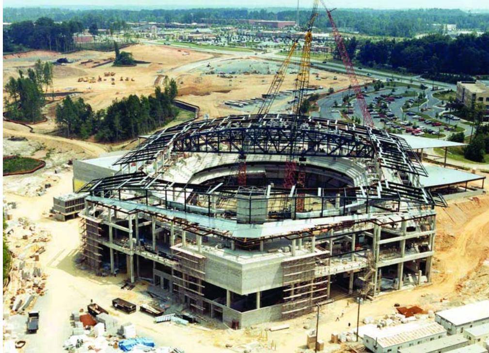
*Above:* The super-trusses exceeded normal shipping sizes. As a result, all connections are bolted so the truss could be assembled in the field. They vary in depth from 12' to 31'. Photo courtesy of Holder Construction
